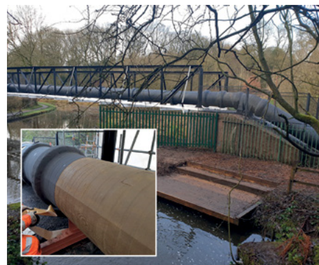
The Steelcoat™ system being applied (inset) and the protected pipebridge.
