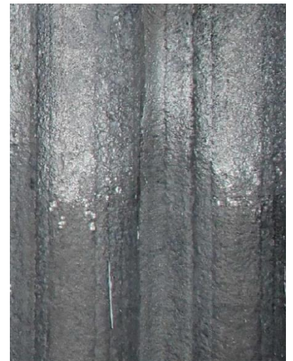
Top half: unprotected Alloy 625 weld overlay section showing wear and degradation.
