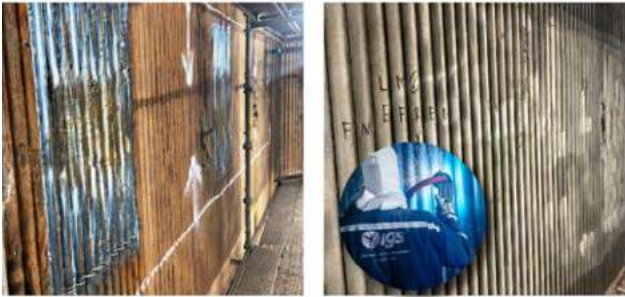
Left - waterwall tubes before surface preparation and the alloy upgrade. Right - waterwall tubes after installation of 5450 HVT alloy cladding
